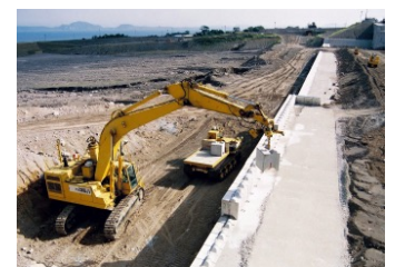
Application to installation of concrete blocks
