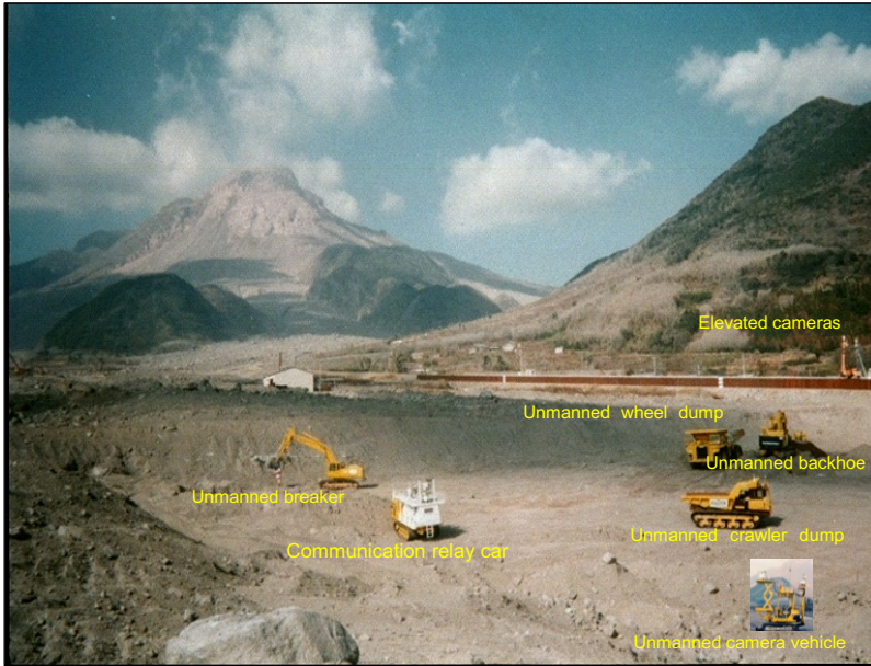
Outline of unmanned construction
